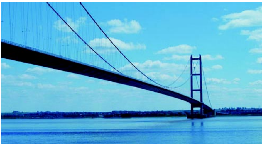
Humberside WSU carries 2 km of Angus Hi-Vol to protect the Humber Bridge
